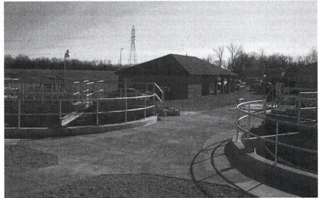
Town of Dillsboro WWTP
