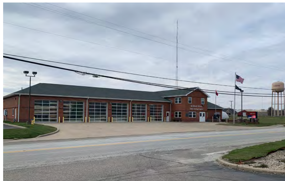
Sunman Rural Fire Department. Source: HWC Engineering
