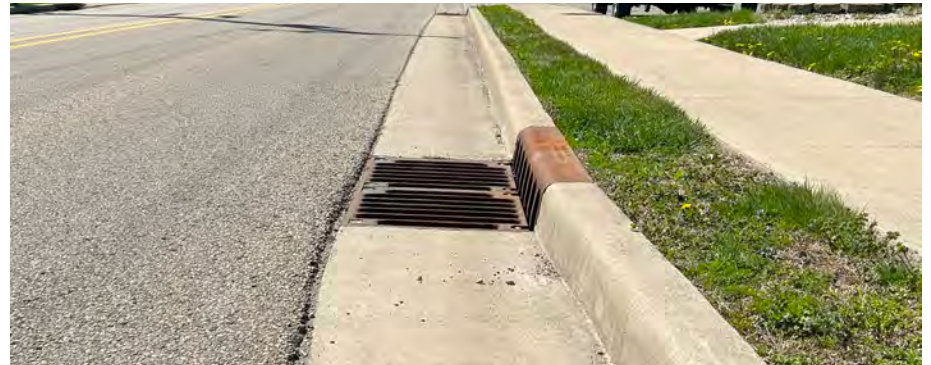
Stormwater drain on Eastern Avenue. Source: HWC Engineering
