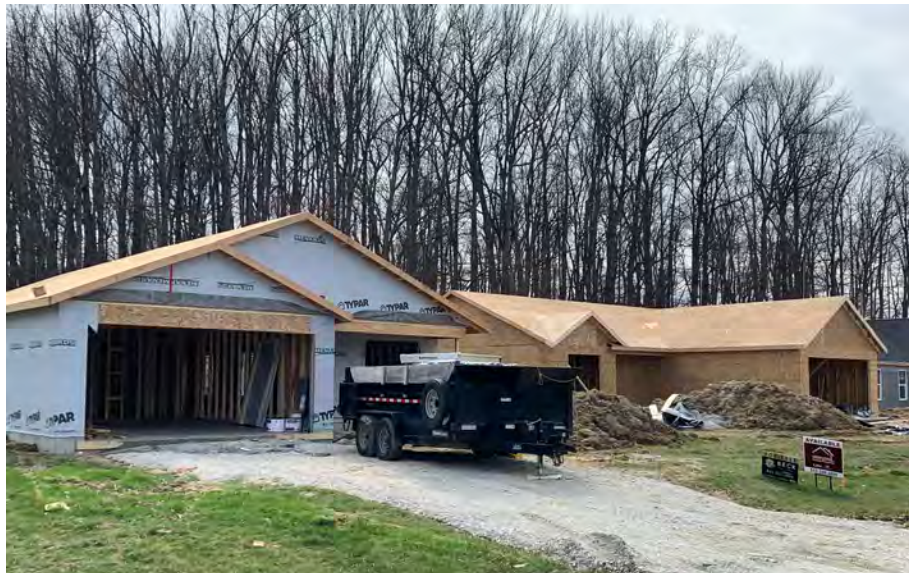
New home construction south of town. Source: HWC Engineering
