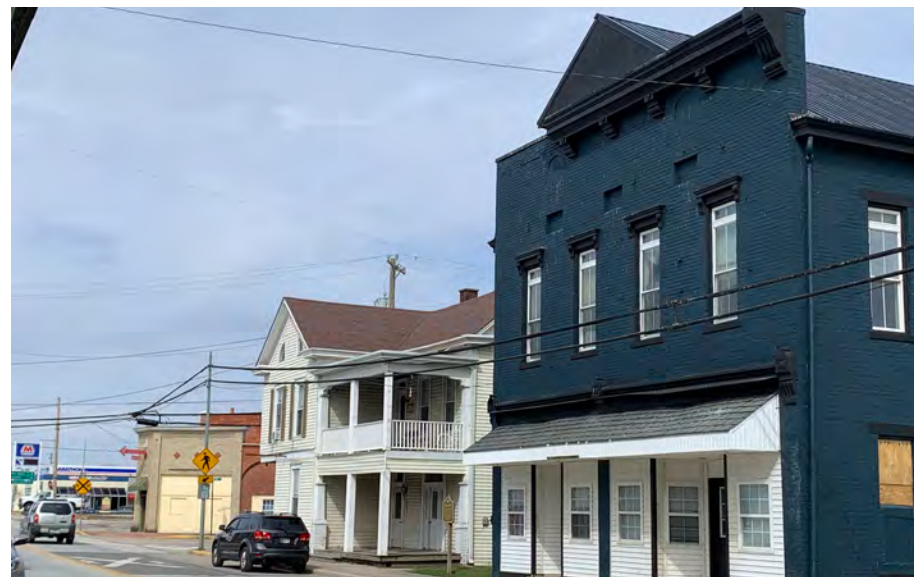
Rehabilitated building on Meridian Street. Source: HWC Engineering
