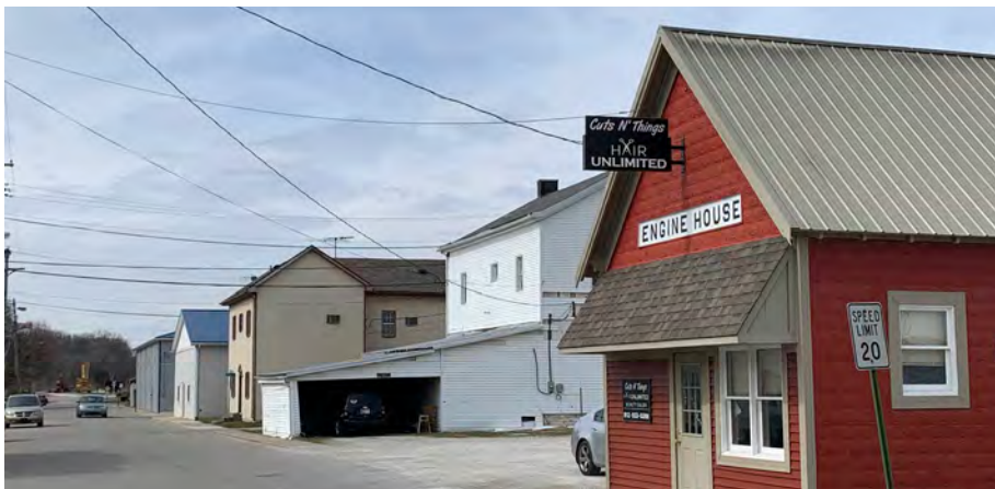
Residential and commercial downtown properties. Source: HWC Engineerings
