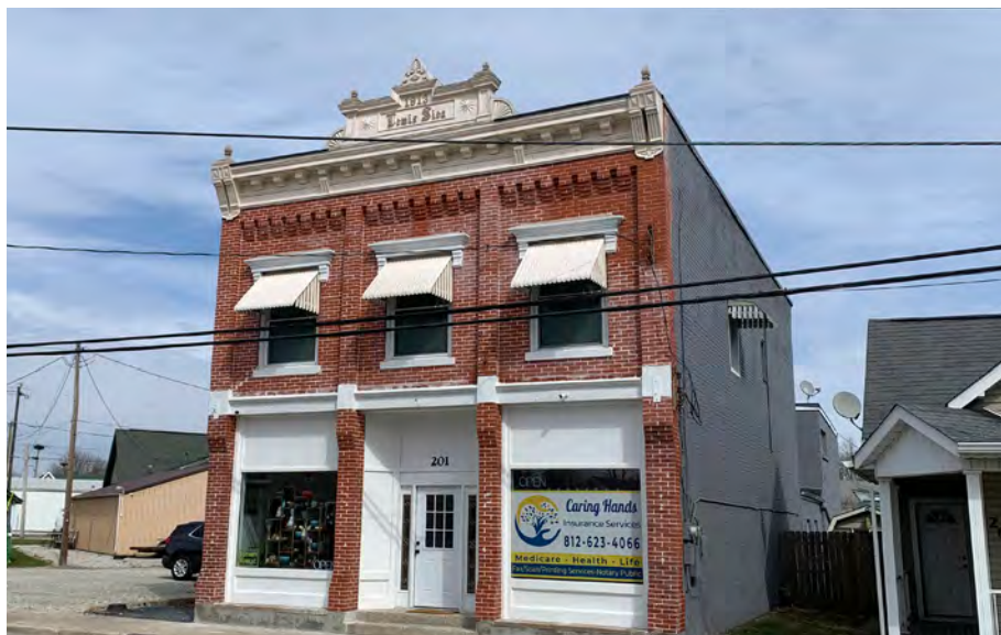
Louis Sieg Building. Source: HWC Engineering
