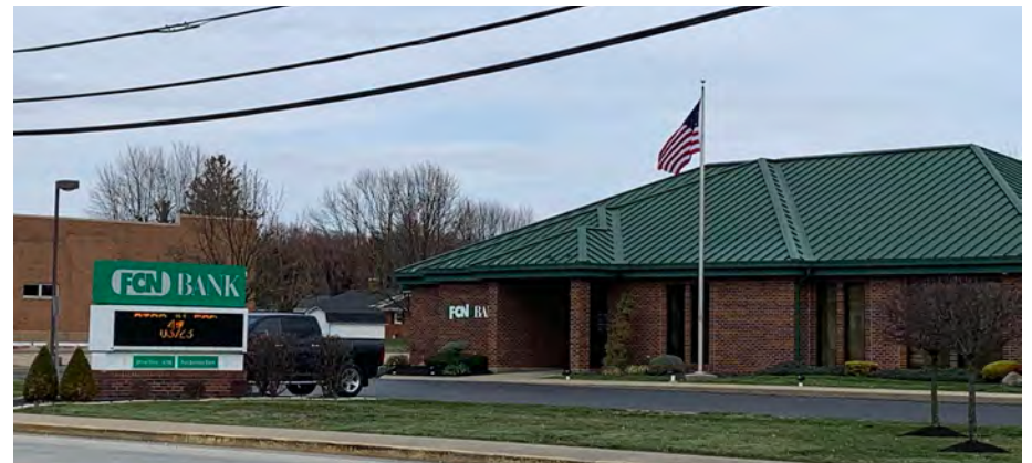
FCU Bank in downtown Sunman. Source: HWC Engineering
