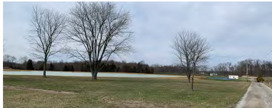
Wastewater treatment plant and settlement lagoon. Source: HWC Engineering
