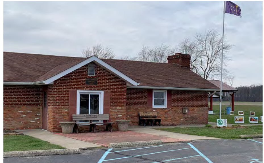
Community building at Sunman Park. Source: HWC Engineering
