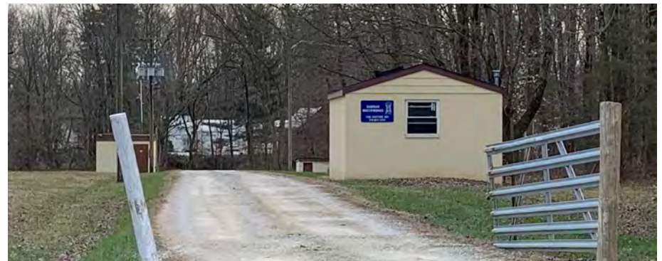
Sunman's water pump station and well field. Source: HWC Engineering
