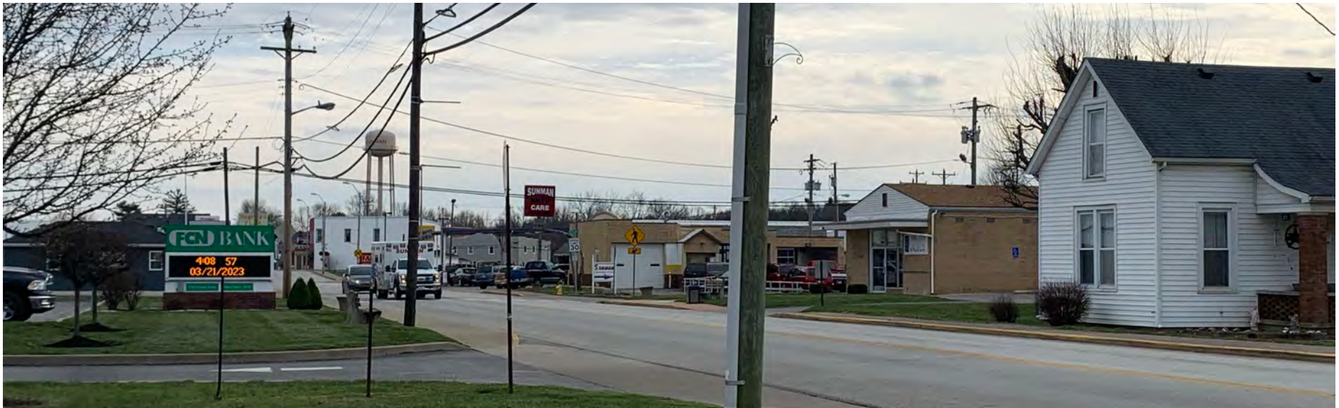
Entering Sunman’s downtown on State Road 101. Source: HWC Engineering
