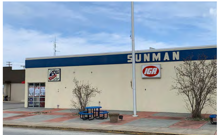
Sunman IGA, the town local grocery store. Source: HWC Engineering
