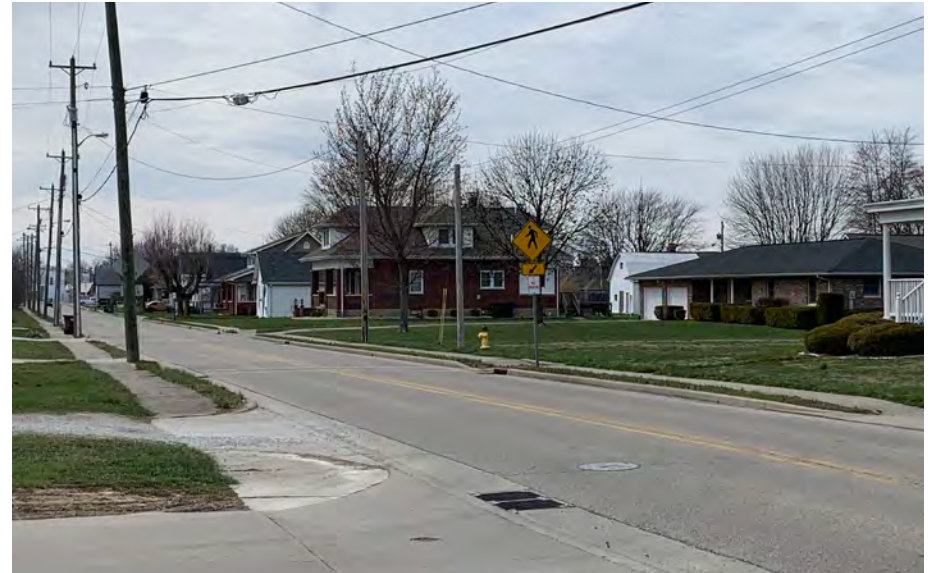
Areas downtown experience flooding during storms. Source: HWC Engineering
